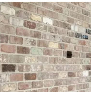
EW-4 EXTERIOR WALL RECYCLED BRICKWORK NAUTILUS
